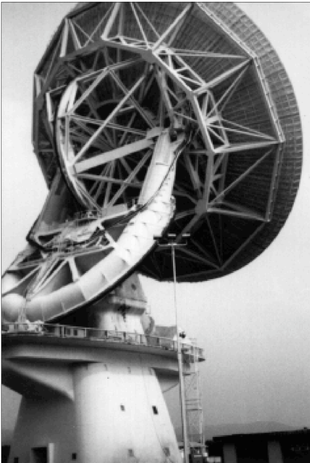
Left: This 140 foot telescope can track the sky with an equatorial mount. The NRAO staff threw a party for it on its 30th birthday.
