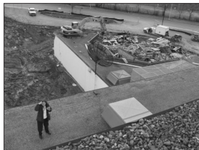
There was stress in January 2007. I can't watch! The old planetarium had to die to build the new one. Photo by Drew Gilmore
