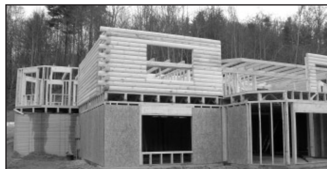
Work continues on our home. The roof and loft area are not yet installed. The turret is on the left side of the image.
